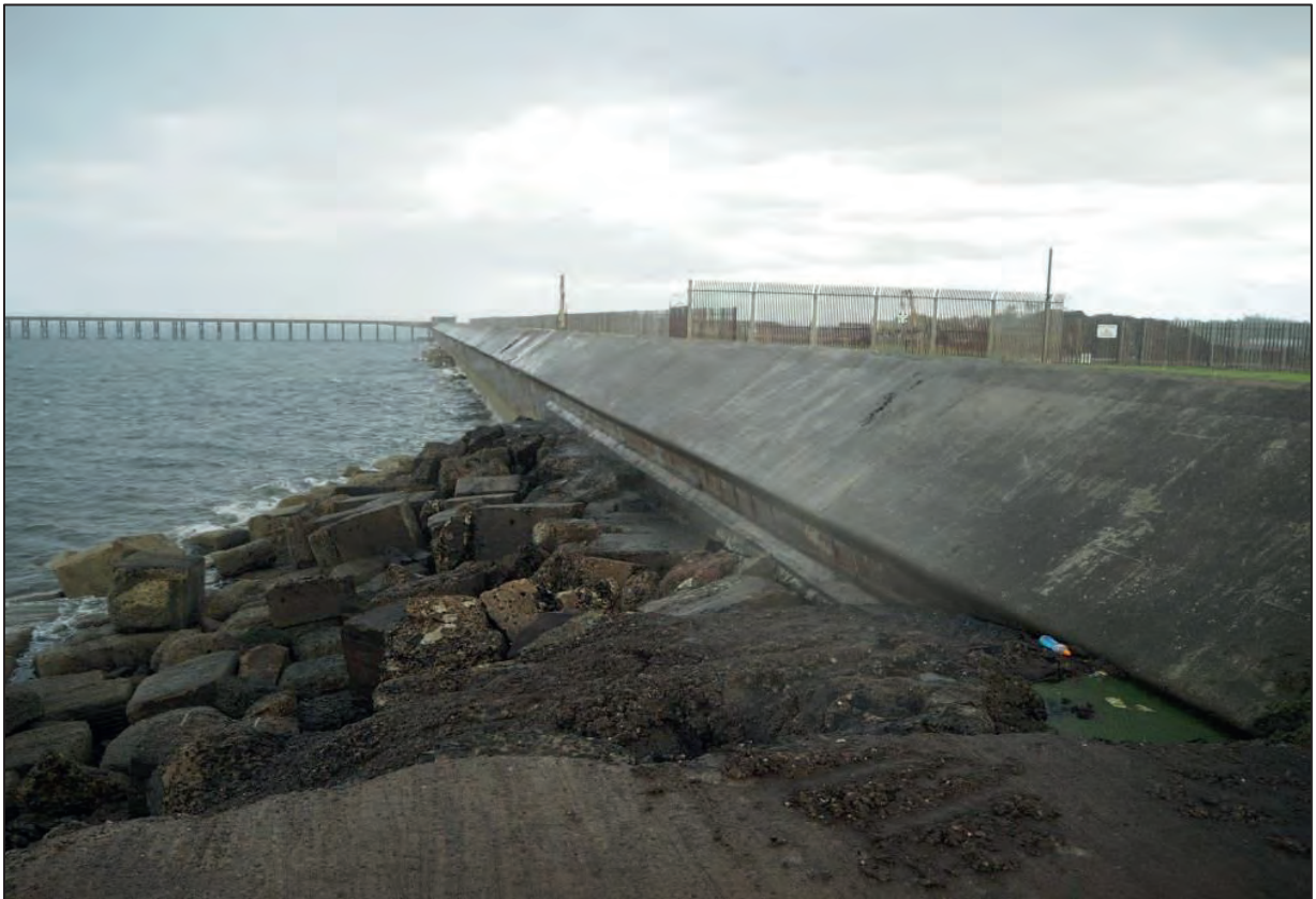
Photograph 07 : Revetment and Seawall
