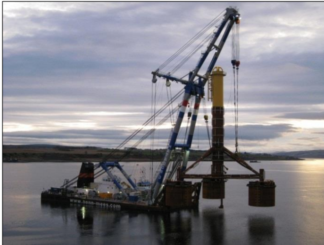
Figure 7.17: An oil and gas platform with suction piles (Source: Ithaca)
