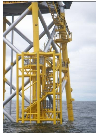
Figure 7.11B: Close up view of the representative WTG Access System (Source : ICOL)
