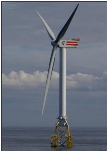
Figure 7.11A: A representative WTG Access System shown on the substructure (Source: ICOL)
