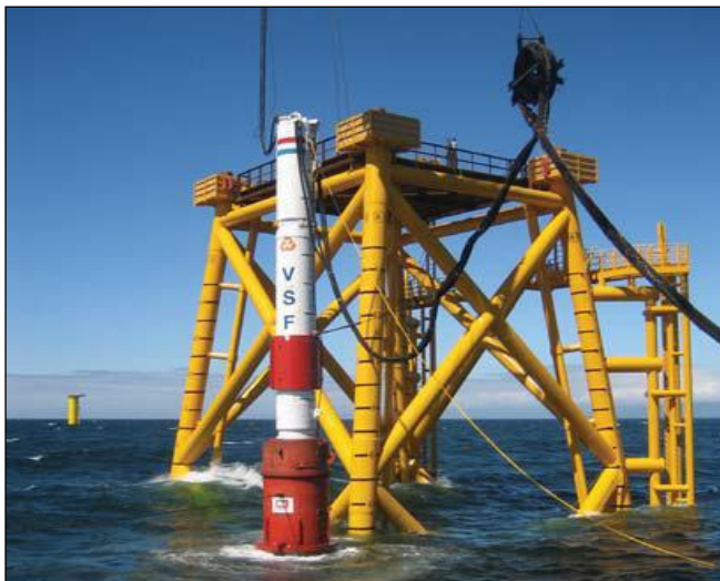
Figure 7.16: A typical pile driving operation (Source: VSF)
